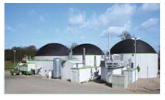
degradation producing methane-rich biogas and the sludge. The biogas production ranges from 50-150m<sup>3</sup>/ ton of wastes, depending upon the composition of waste. The biogas can be utilised either for cooking/ heating applications, or through dual fuel or gas engines or gas / steam turbines for generating motive power or electricity. The sludge from anaerobic digestion, after stabilisation, can be used as a soil
